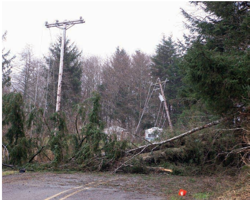
Disrupted distribution lines
