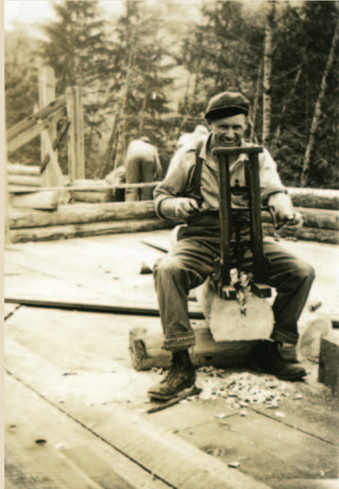
Cabin construction without electricity, 1948.
