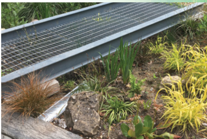
Rain gardens channel rain into a shallow planted depression to allow the water to soak into soil. Featured rain garden by wendyallendesigns.co.uk
